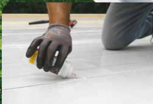
*Easily seal T-joints and edges with Leadax Liquid PVB*
